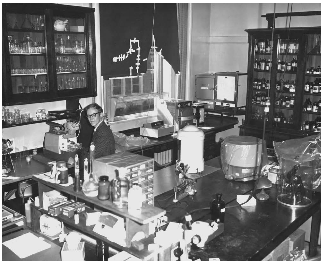
Laboratory, second floor, C-wing, Sterling Hall of Medicine c1969. Thomas L. Lentz at Porter-Blum ultramicrotome used for making thin sections for electron microscopy. This was the state of laboratories at the time, prior to the renovations for the new Section of Cell Biology.
